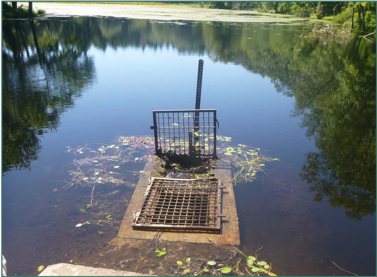
Drop Inlet Type Structure, Photo Taken August 5, 2013, by RTG
